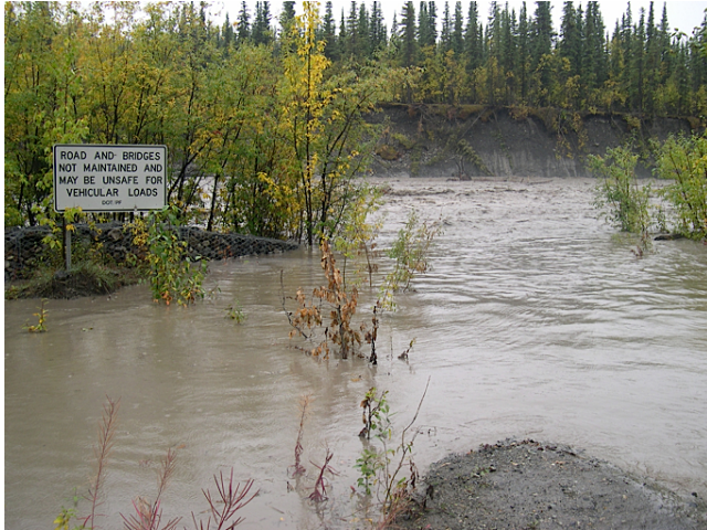
Photo 3: Access bridges to McCarthy area often wiped out by flooding and erosion, 2007.
