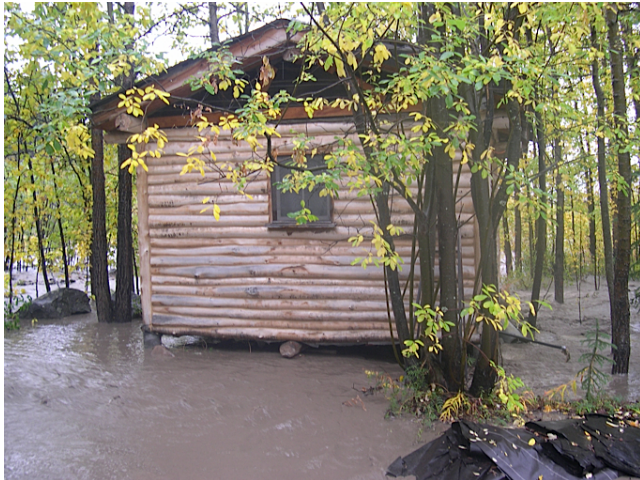
Photo 1: McCarthy Creek flooding just downstream from the footbridge, 2007.
